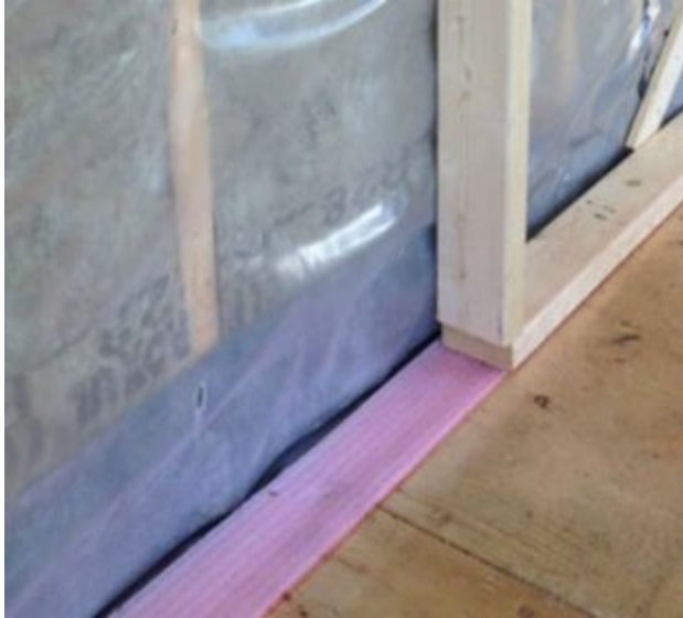
Double wall assembly © Bala Structures
